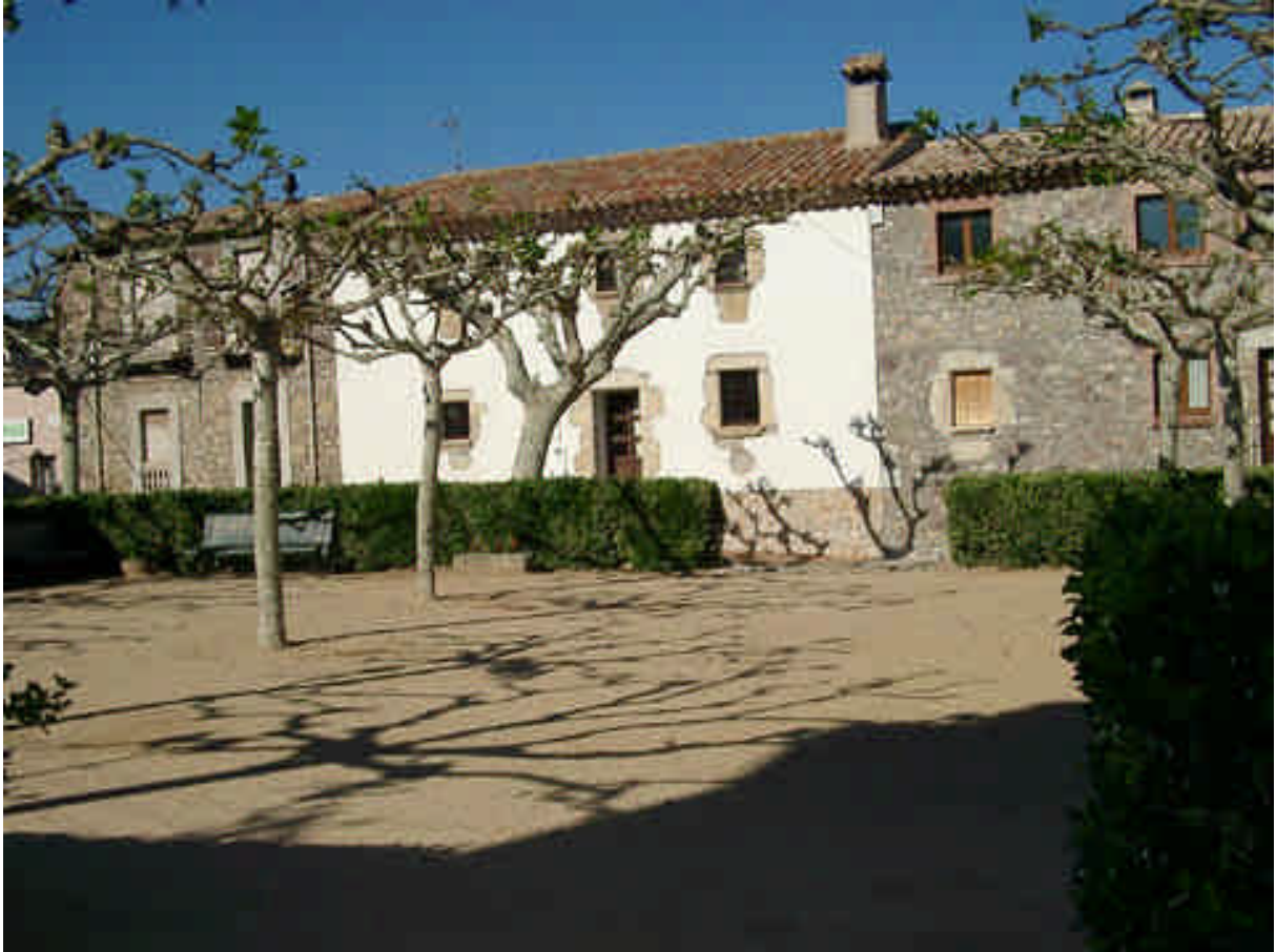
Image 1: Western view of the house
